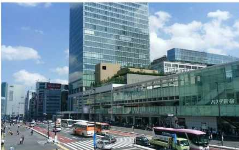
Toyo/Red-White's Valves Are used on High-rise buildings at Shinjuku, Tokyo Metropolitan Subcenter
